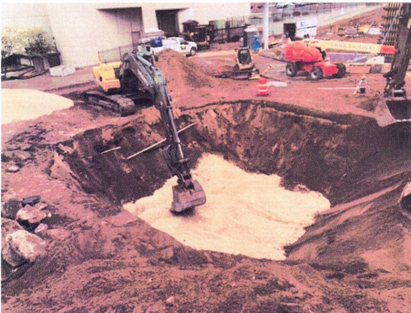
Approximately 2' of clear rock placed before soil backfill at gridlines 2.3/D
