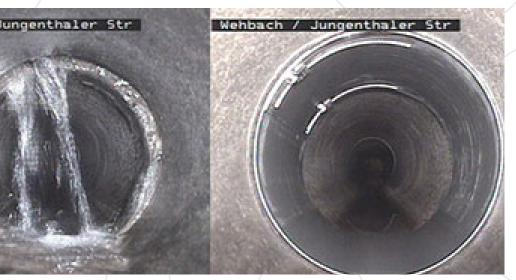
Sleeve Sizes are Available from 6" to 32" in Circular Pipe Diameter QuickLock is a strictly mechanical point repair system for the inside repair of pipes.
