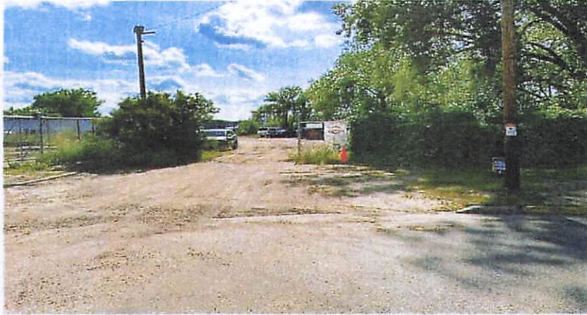
Figure 2 - Parcel Entrance on 7/19/23. Fencing and Gate would be Removed and Replaced
