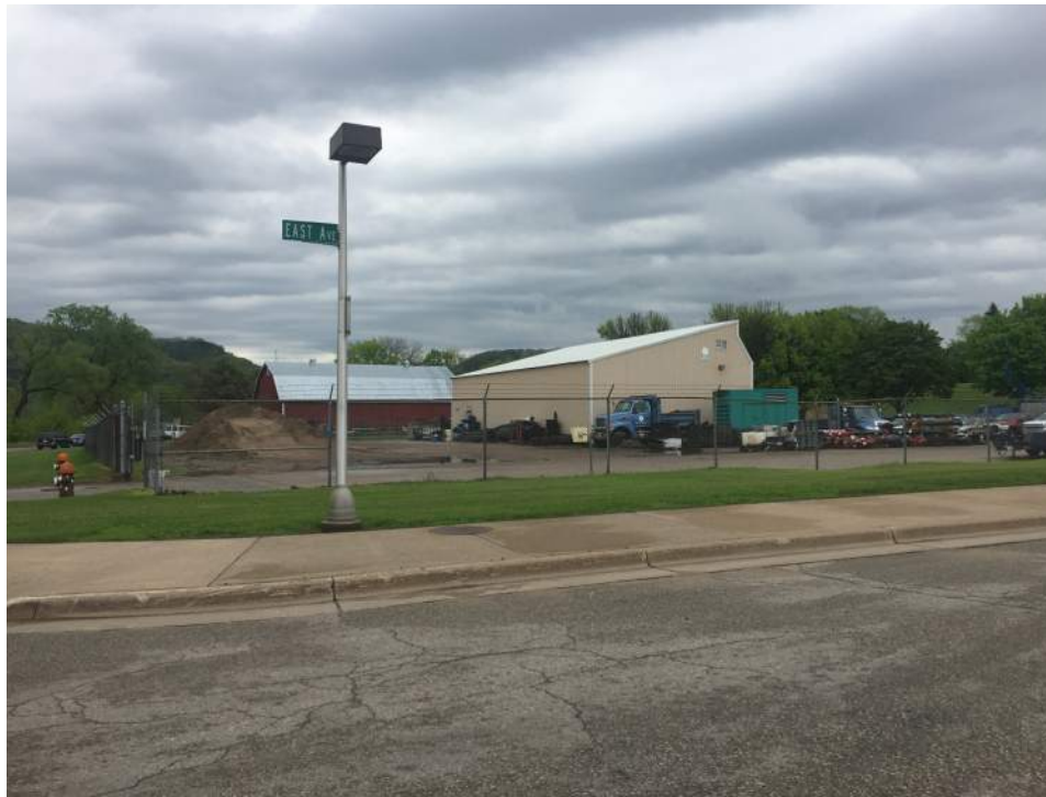
ENTRY TO EXISTING SITE OFF EAST AVE
