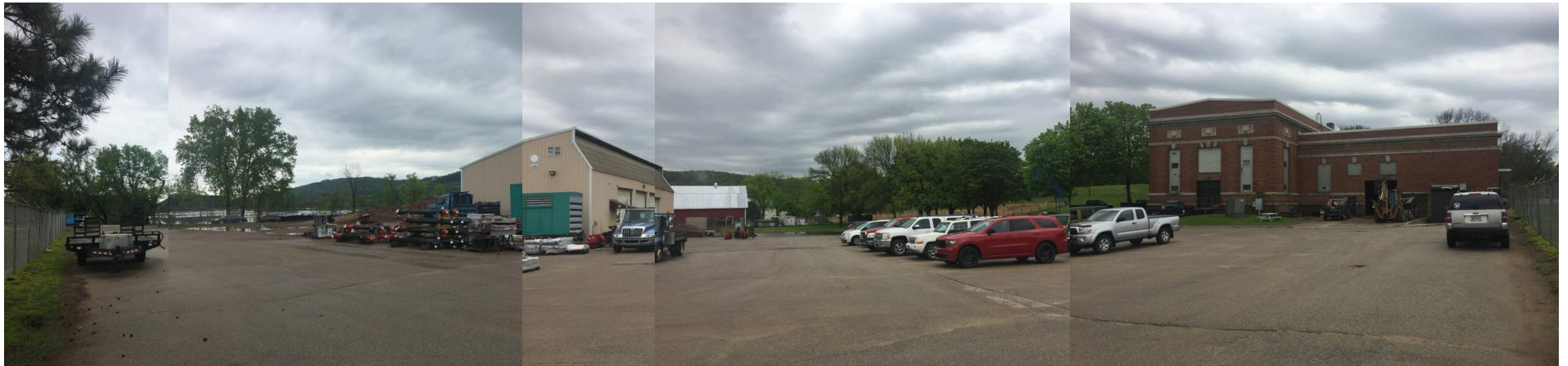
EXISTING LAX UTILITY SITE OVERVIEW FROM NORTH TO SOUTH
