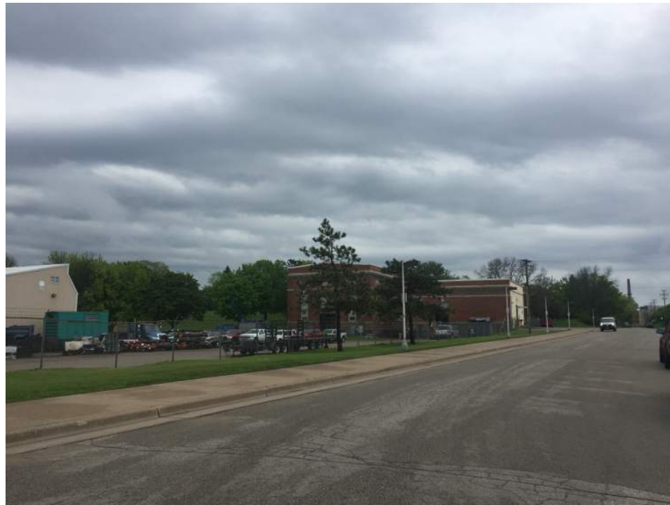
EXISTING LAX UTILITY SITE FROM EAST AVE
