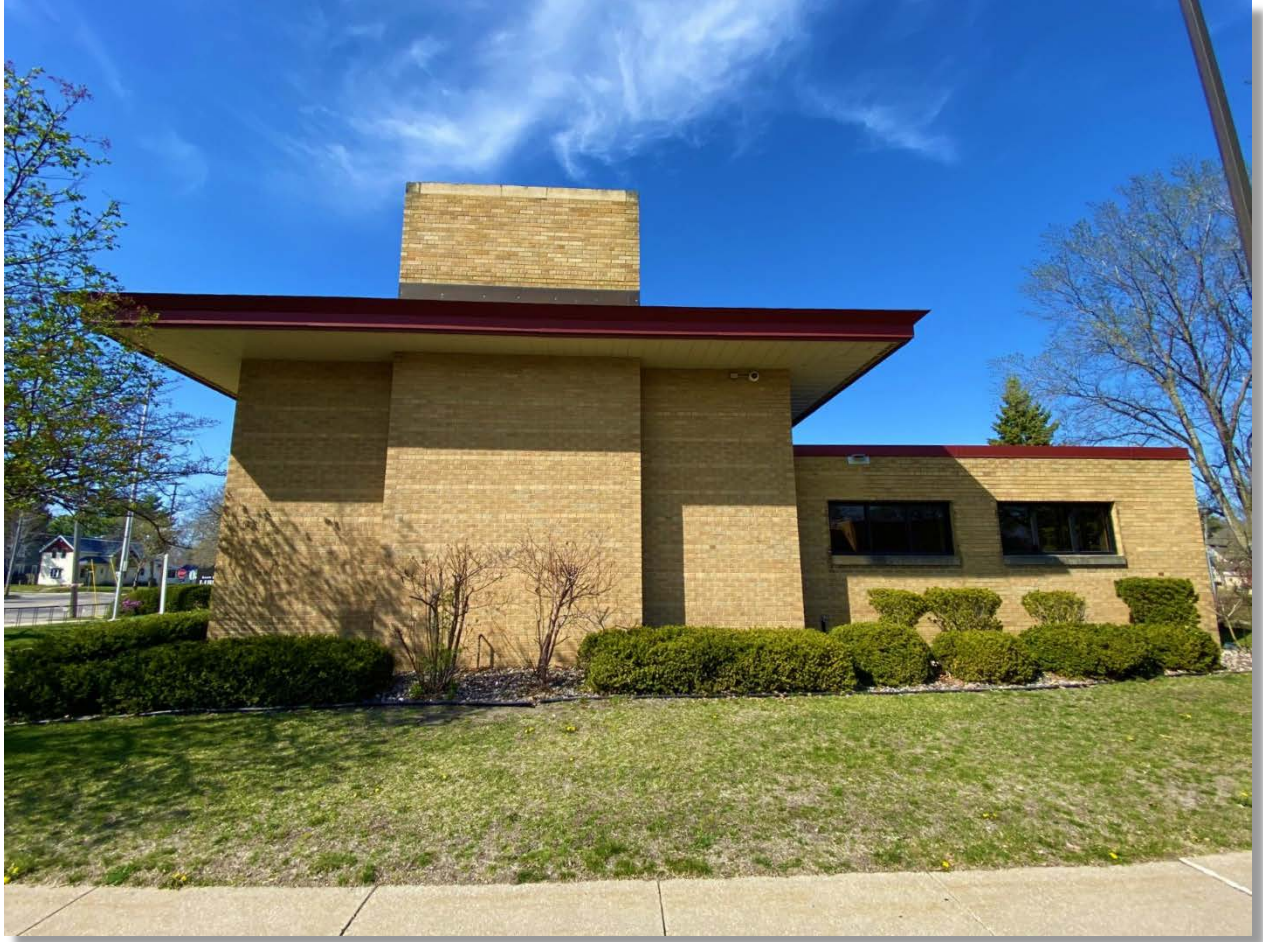
South Branch Library, South Elevation, 2024. Source: David Riel.
