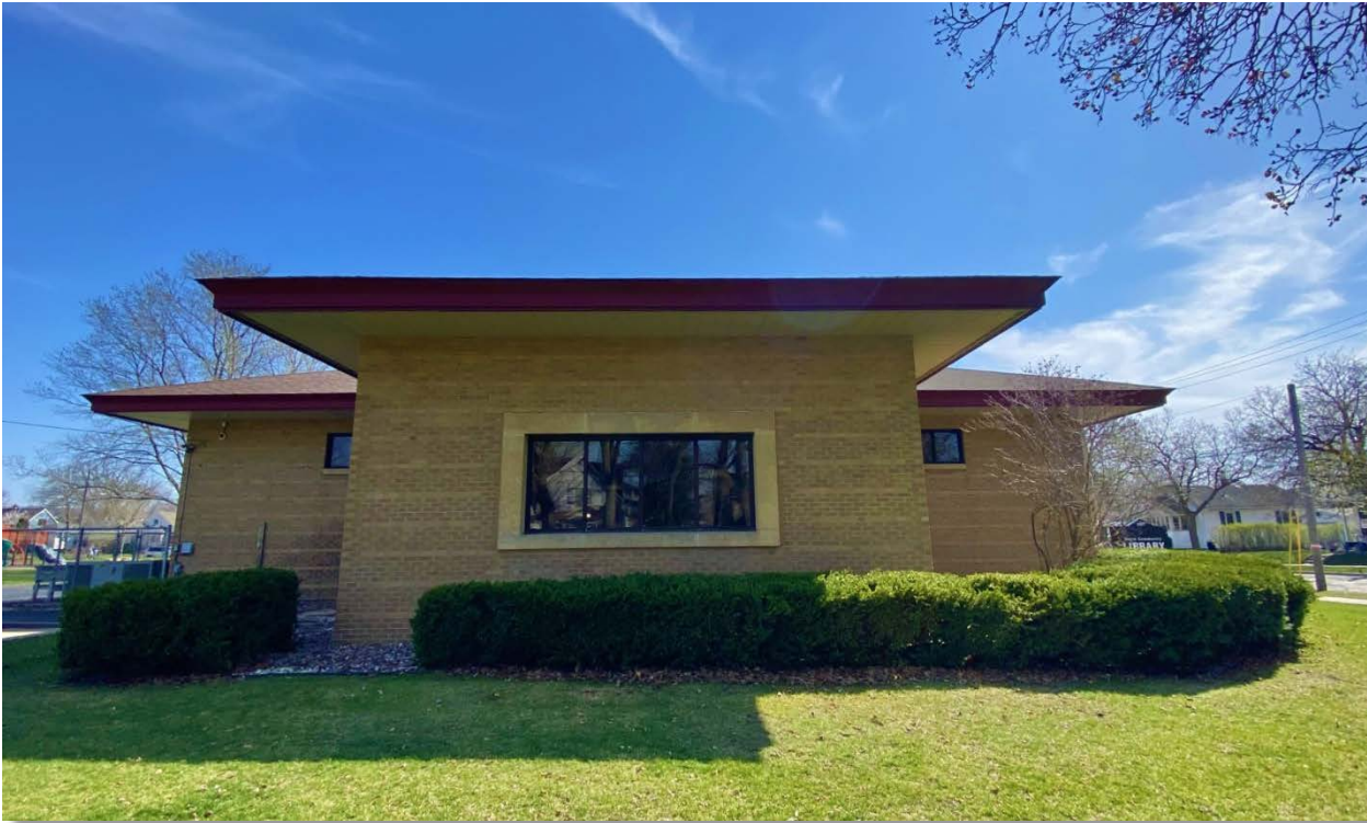
South Branch Library, North Elevation, 2024. Source: David Riel.
