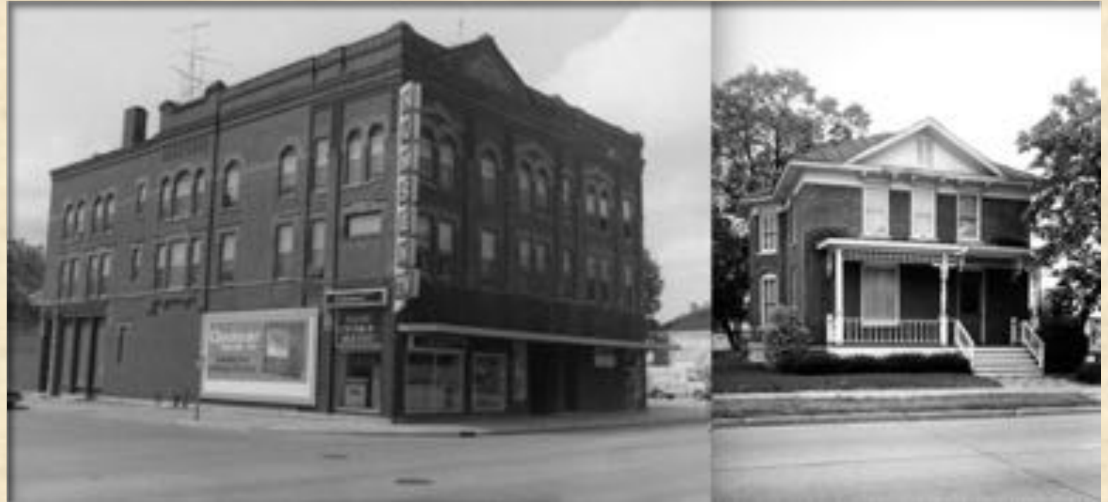
J.P. Koller Building (Left). John Halverson House (Right). Ca. 1977. Source: Wisconsin Historical Society.
