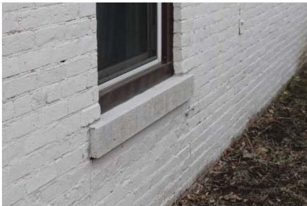
New stone sill in painted brick wall. (2012)
