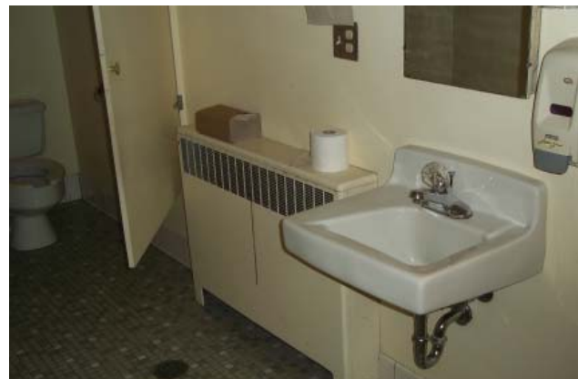
Second floor Women's restroom sink. (2012)
