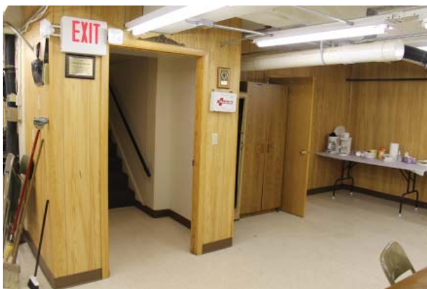
Central egress stair from basement. (2012)
