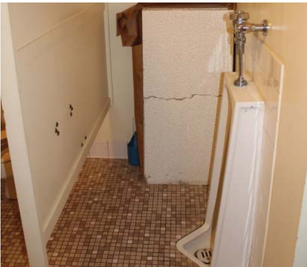
Men's room used for building material storage. (2012)
