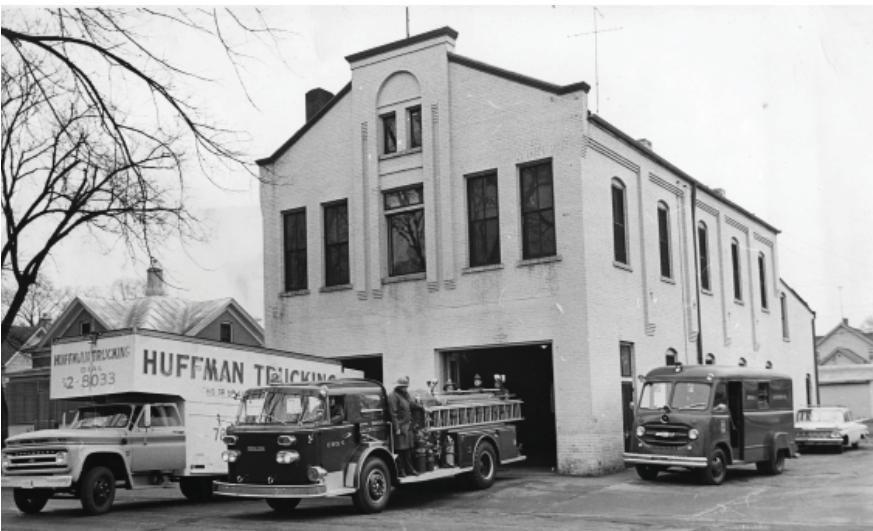
Fire Station #5 (c.1960)
