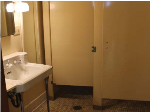
Out-dated and inaccessible first floor restrooms. (2012)
