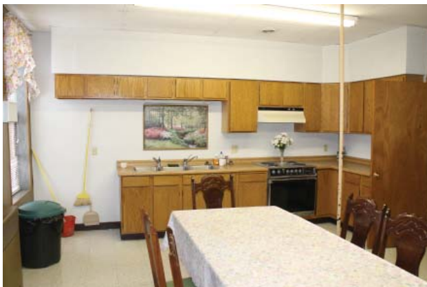
Second floor kitchen with vertical tie rod. (2012)
