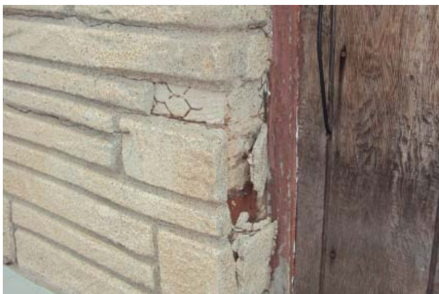
"Stone" patterned stucco on main facade. (2012)
