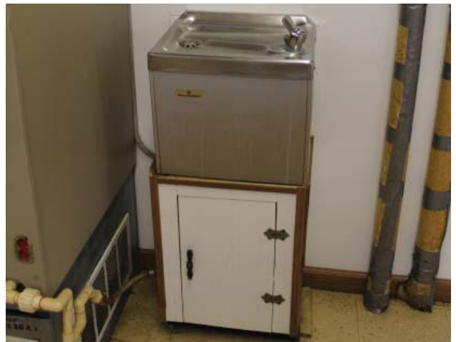
Inaccessible drinking fountain. (2012)
