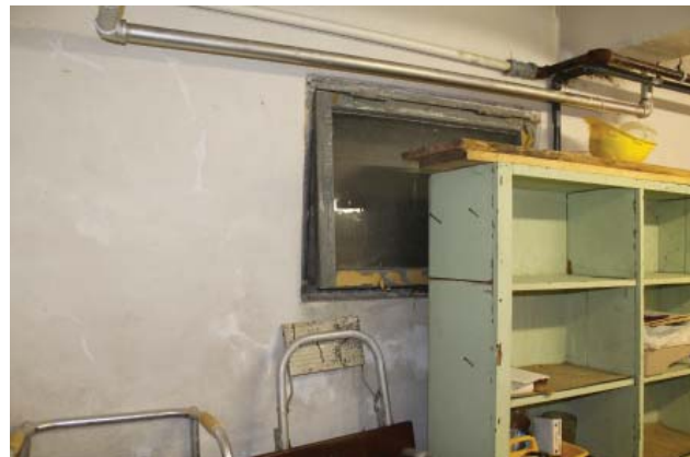
South west storage room, exterior window. (2012)
