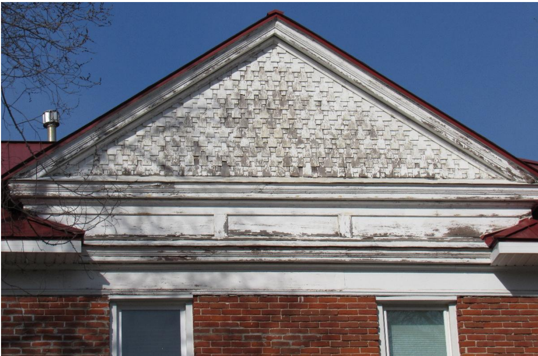
Figure 13 – Detailed view of front gable with wood shingles. March 2026.
