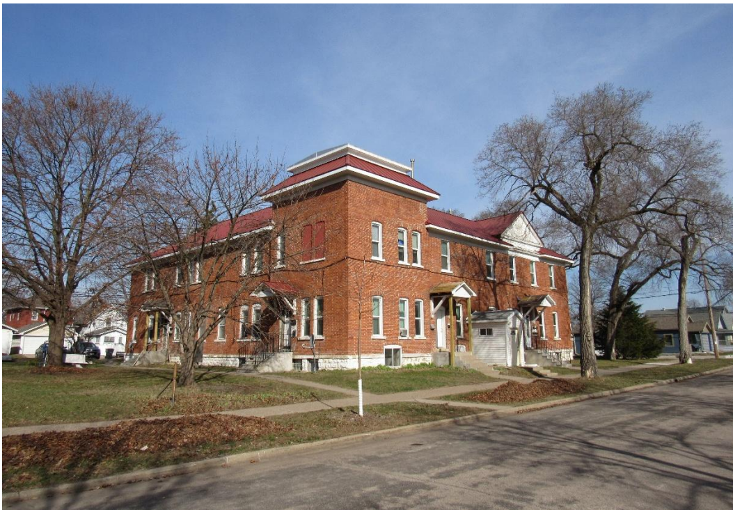
Figure 15 – View of the south and east elevations of the Goddard Hotel, taken from Prospect Street. March 2026.
