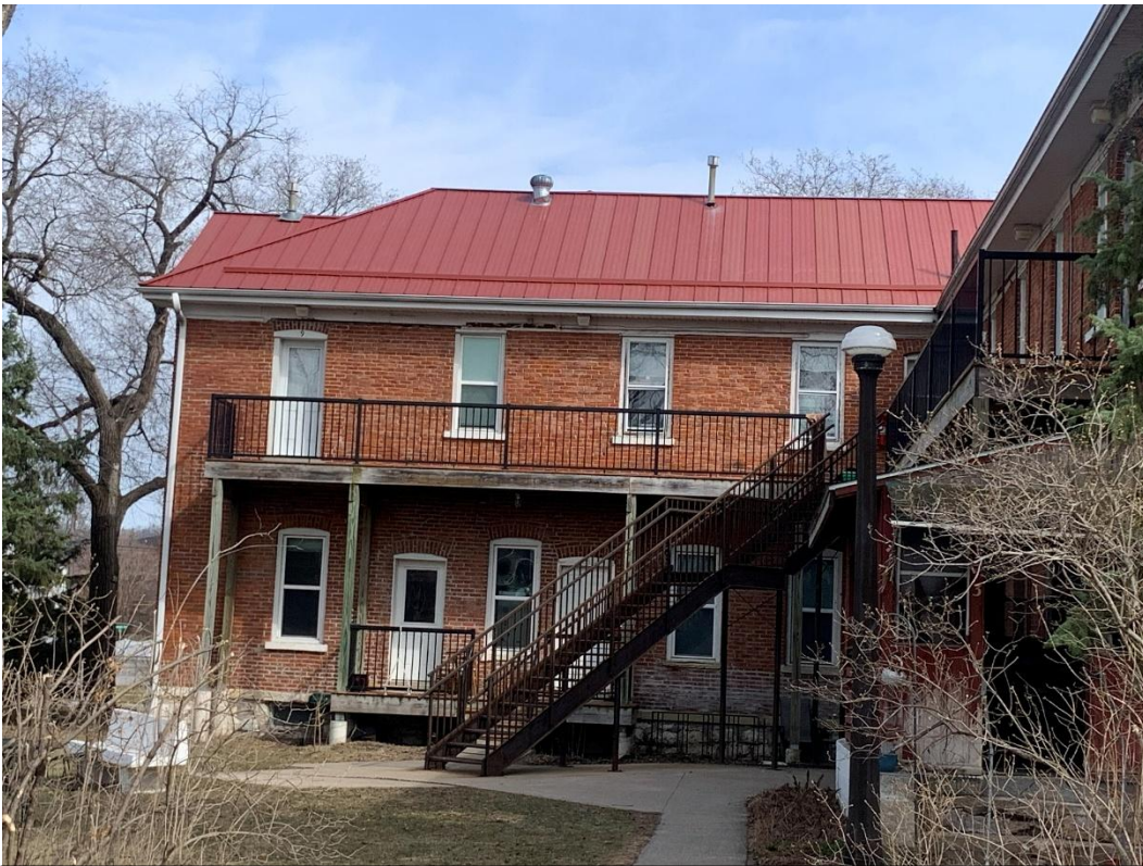
Figure 19 – View of the west façade of the hotel addition. March 2026.
