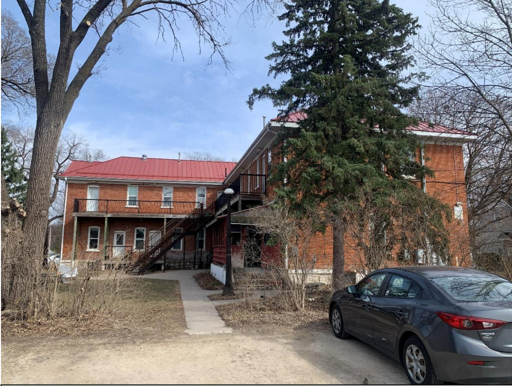
Figure 20 – View of the west façade of the Goddard Hotel. March 2026.
