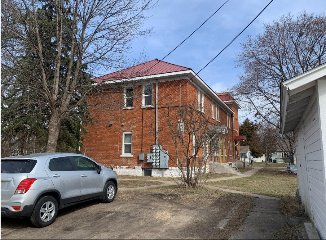
Figure 18 – View of the west façade of the original hotel. March 2026.
