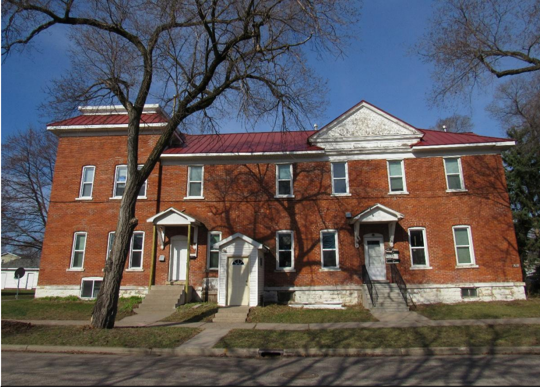
Figure 12 – View of east (front) façade of Goddard Hotel. March 2026.
