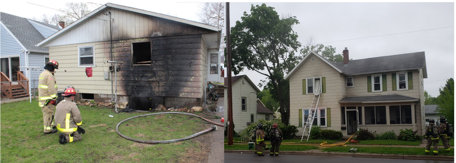
2022 Investigated Fire Incidents
