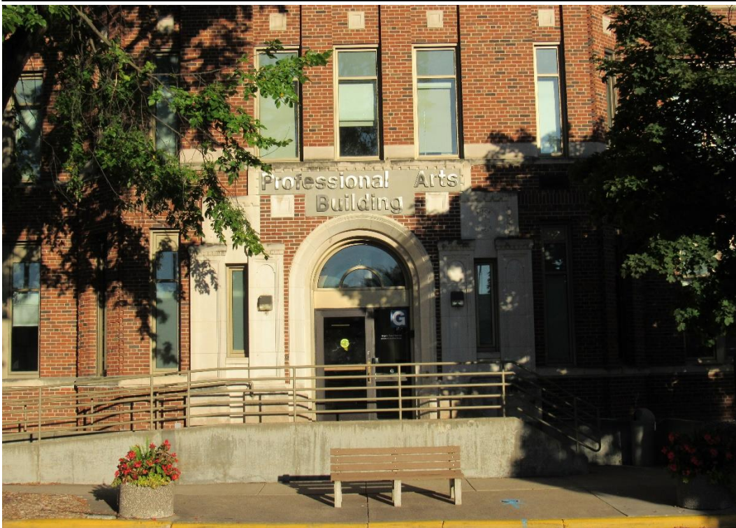
Figure 14 – Detailed view of west (front) façade of School of Nursing. October 2025.
