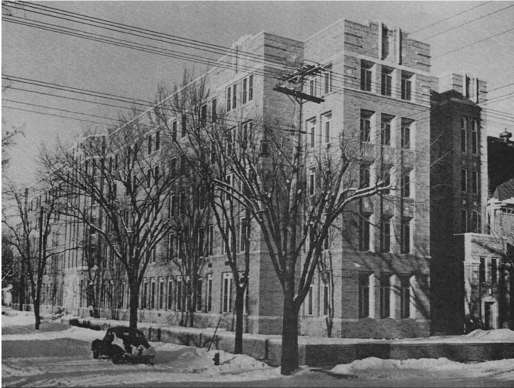
Figure 7 – View from 10 th and Market Streets looking northeast at St. Francis School of Nursing Ca. 1943. Courtesy of La Crosse Public Library Archives.
