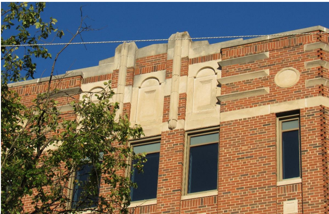
Figure 16 – Detailed view of the parapet detail above the main entry at the School of Nursing. October 2025.
