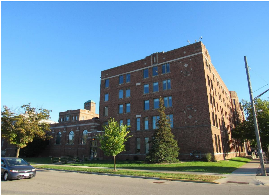
Figure 20 – View of the north façade of the School of Nursing. October 2025.
