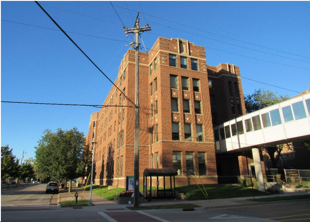
Figure 17 – View of the south façade at the School of Nursing. October 2025.
