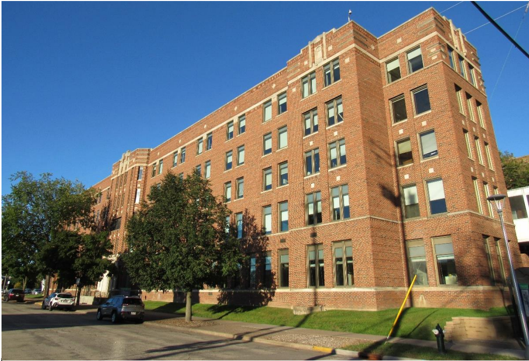
Figure 13 – View of west (front) façade of School of Nursing. October 2025.
