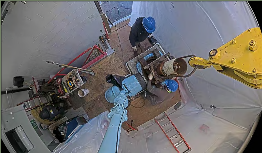
Well 16 Pump Being Pulled in 2025
