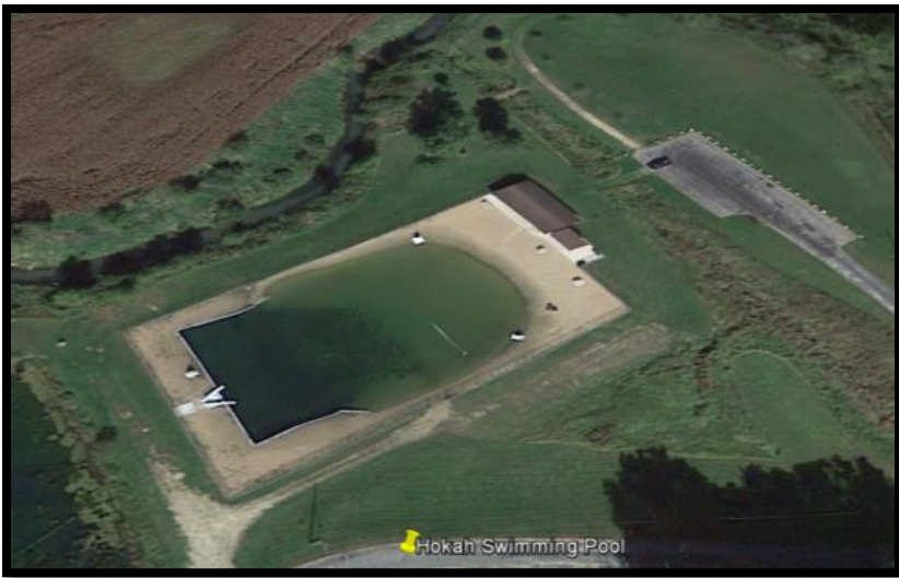
Hokah Swimming Pool- Hokah, MN
