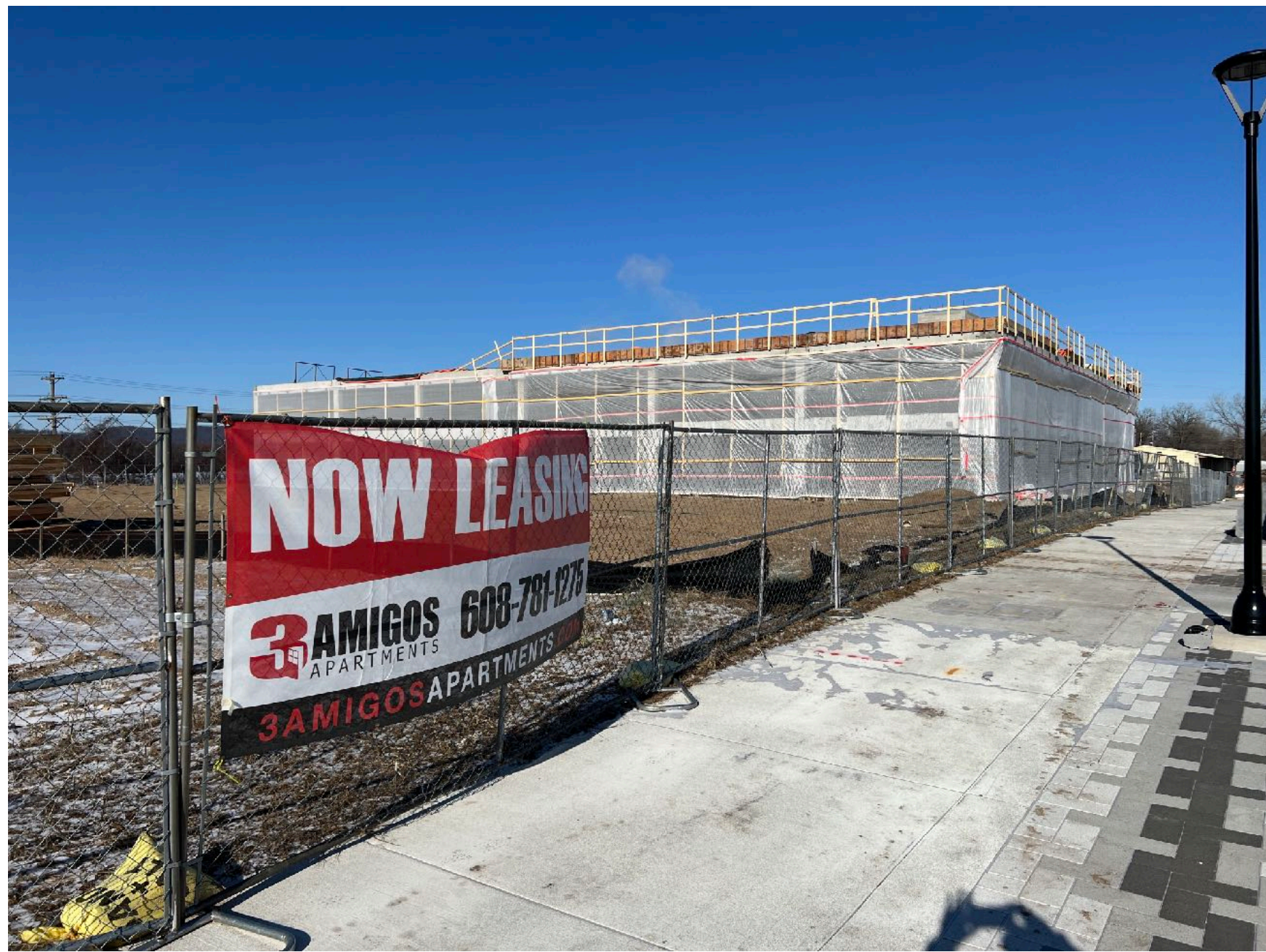
Progress on War Eagle, January 15, 2025
