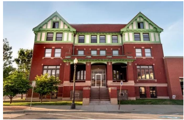
Pomeroy Properties. 1913 Apartment Restoration Progresses. https://www.pomeroypropertiesks.com/post/1913-apartment-restoration-progresses
