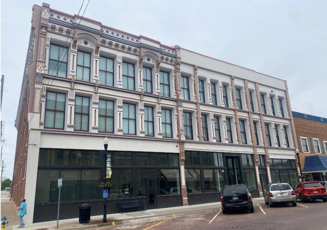
Figure A.1 – Union Lofts – 20 South Main Street in Fort Scott
