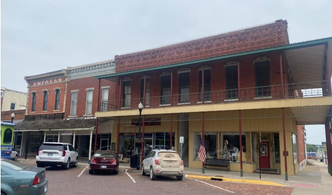
Figure A.3 – East side of North Main Street, bordering East Wall Street in Fort Scott
