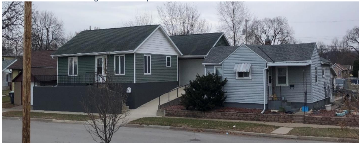
Figure 17: Examples of Elevated Home in La Crosse
