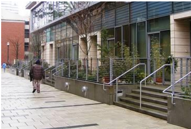
Ground floor units with separate entrances
