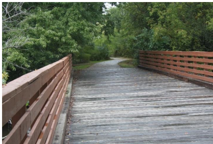
Existing Pedestrian Bridge
