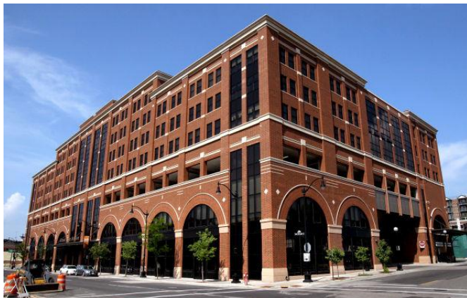
Photo: The Grand River Station downtown houses the La Crosse Transit Center
