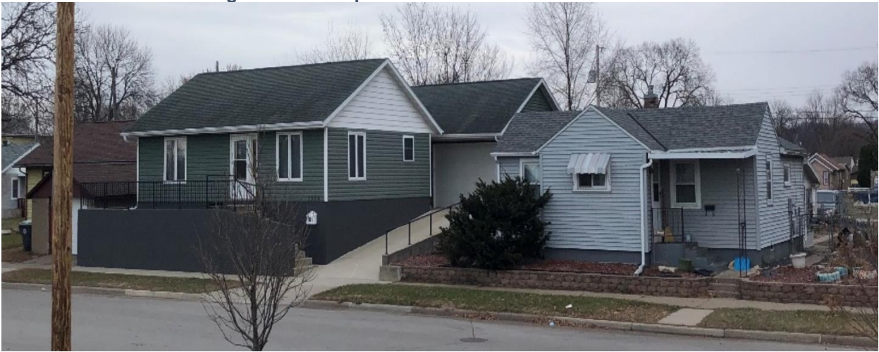
Figure 17: Examples of Elevated Home in La Crosse
