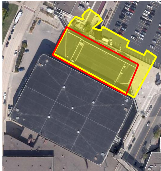
Fort Smith Performing Arts Center (Fort Smith, AR) 1,300 seats
