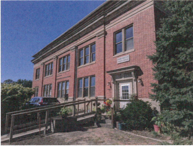
Front of building
