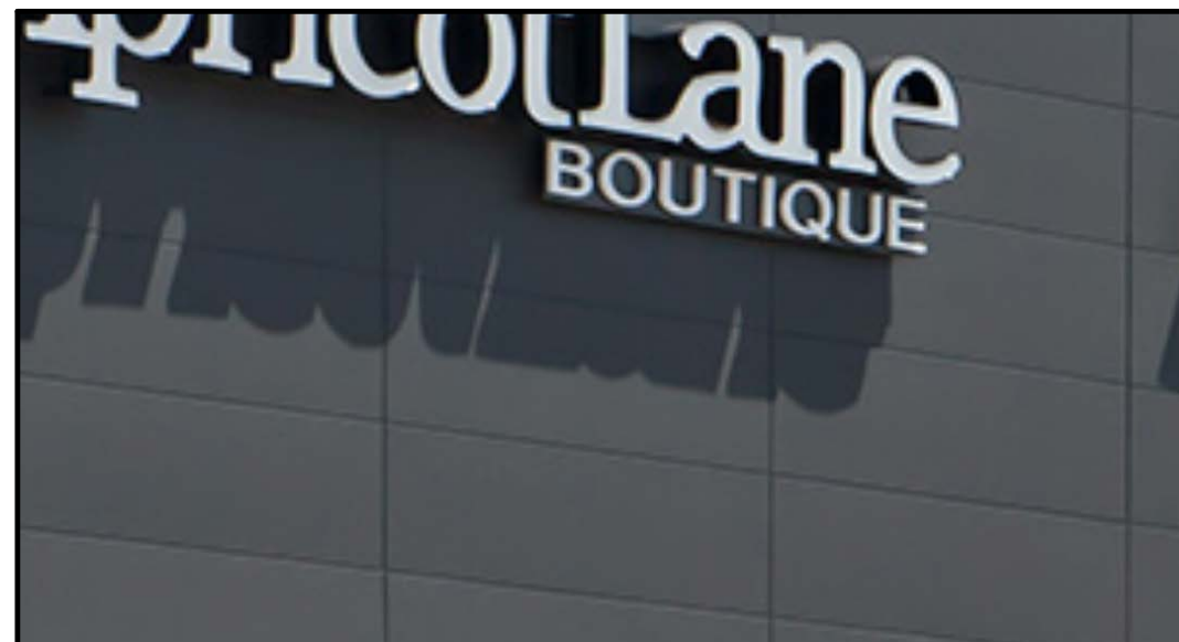
FIBER CEMENT PANEL SIDING - BRK-1
