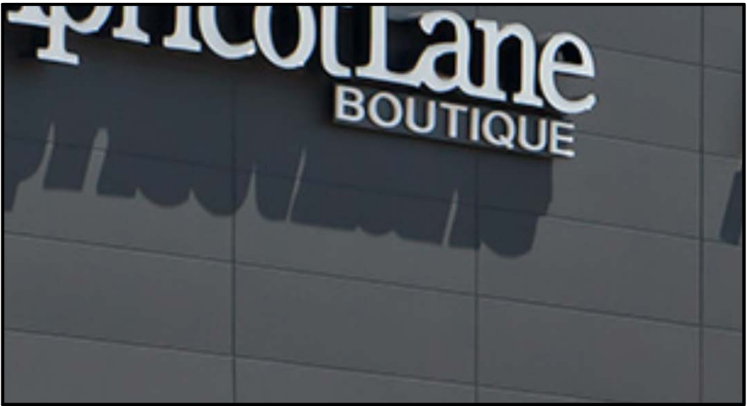
FIBER CEMENT PANEL SIDING - BRK-1 BRAND: NICHHA COLOR: STEELE FINISH: TUFFBLOCK
