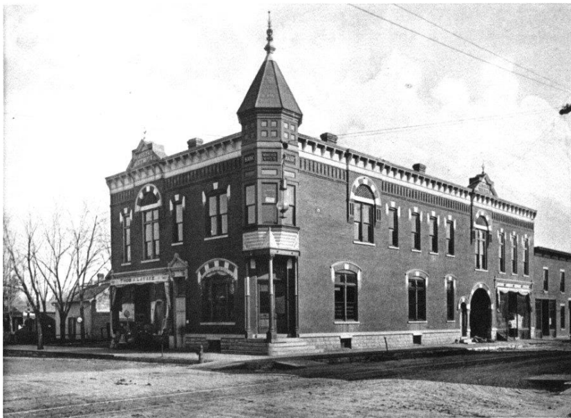
THE EXCHANGE STATE BANK (NORTH SIDE.)
