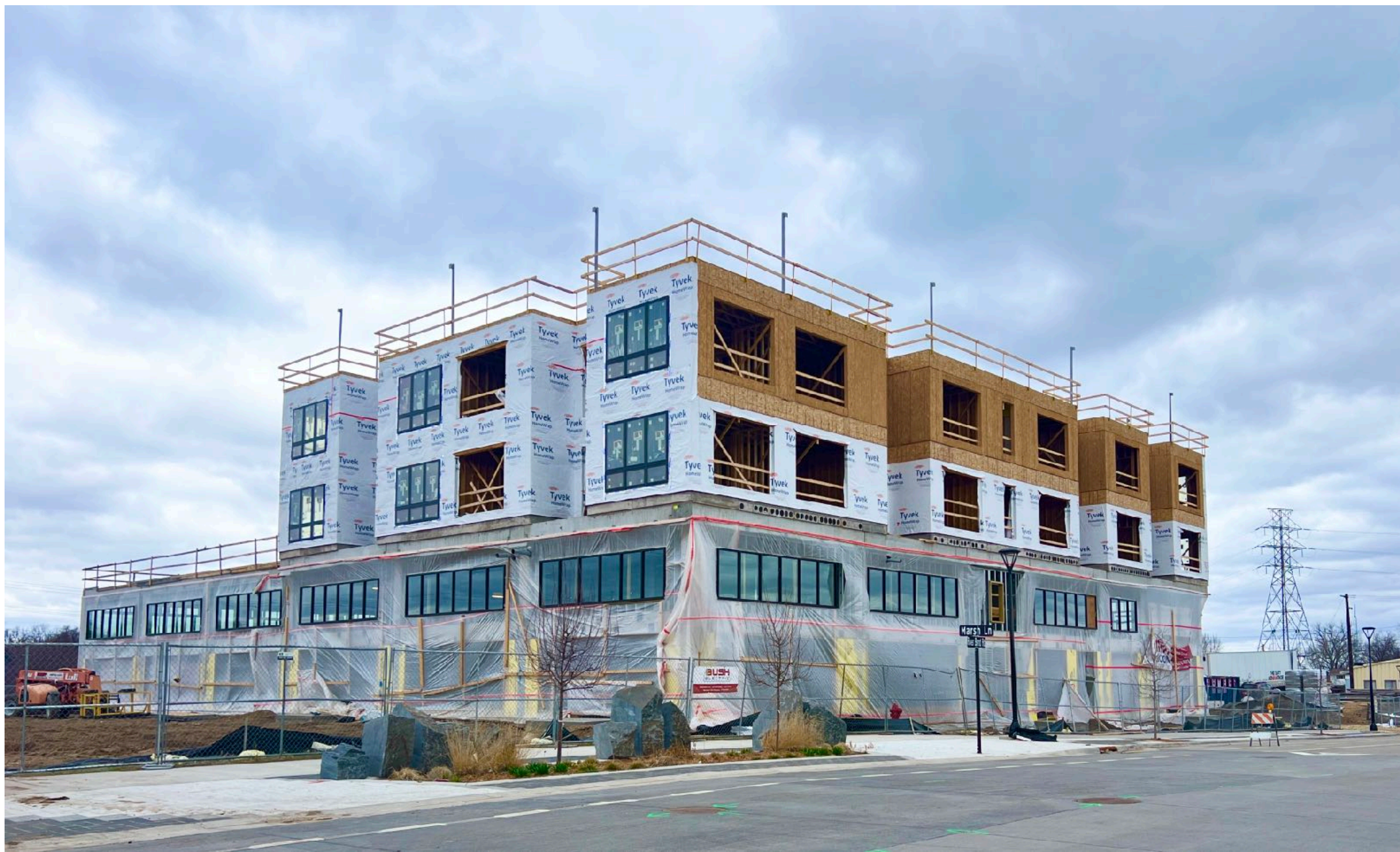
Progress on War Eagle, April, 2025
