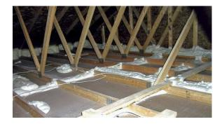
For homes with "kneewall" attics, triangular crawlspace style attics usually on the 2<sup>nd</sup> floor of a home against a living space, care must be taken to ensure proper air seal and insulation. It is possible to insulate either the roofline <u>or</u> the wall <u>and</u> floor. Be sure to properly air seal around the entrance, electrical boxes, pipes, etc.
