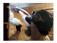
Two-part spray foam, or rigid foam sealed at the sides with one-part spray foam or caulk, both insulates in a thin portion of your building's envelope, as seals air leaks to outside. By definition, rim joists are above ground and can lose a lot of heat while causing moisture concerns.
