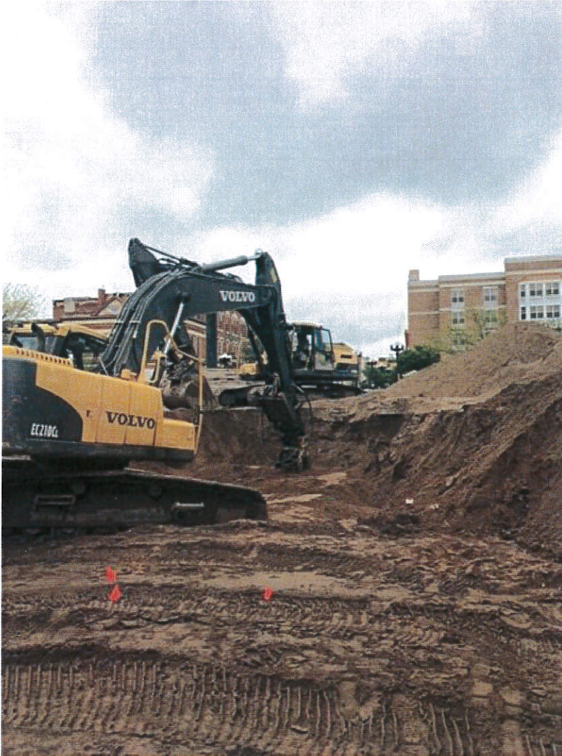
Overdig excavation
