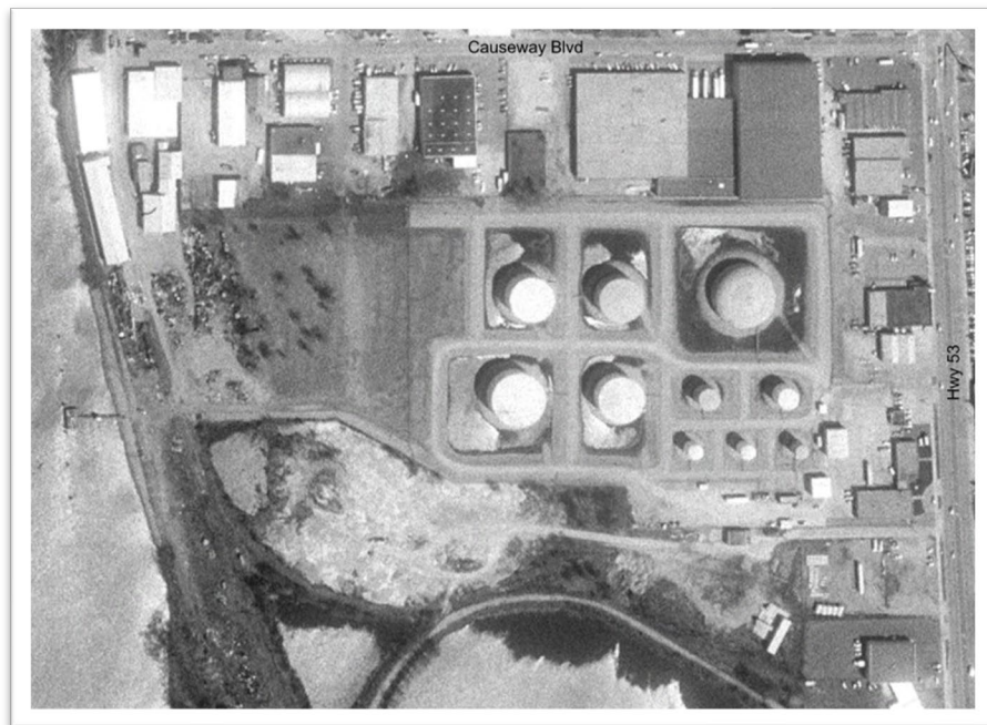
1992 Google Earth image of the project site.
