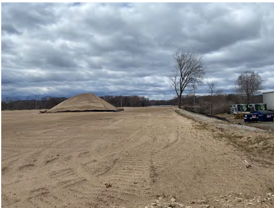
Photo 3 Near Kraft Street, looking west.
