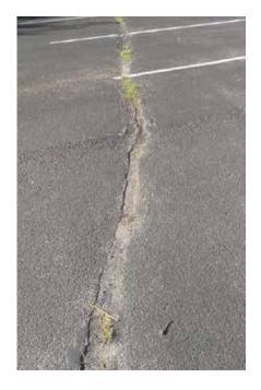
The paved area immediately adjacent to the southeast door of the art room has depressed significantly, leaving the transition threshold a difference of
