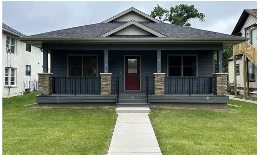
After New Construction
