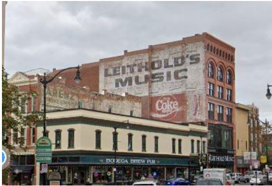
Leithold Music Building & Jules Buildings (116 4 th Street S & 327 Pearl Street)
