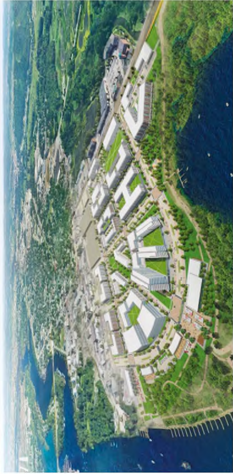
6.5 Aerial Image Aerial looking north east capturing the River Point District's overall scale and relationship to the existing natural landscape.
