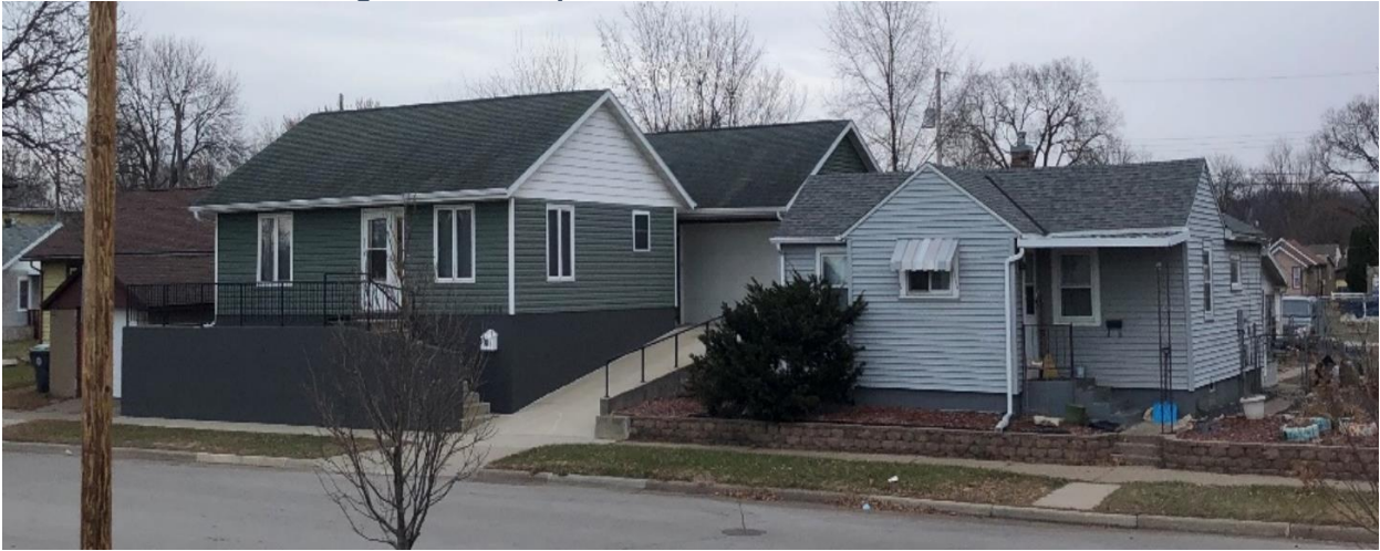
Figure 17: Examples of Elevated Home in La Crosse
