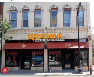
The Pearl Street wall sign will be 2'-0" in height and 9'-5" in width. It consists of black aluminum panels with a translucent acrylic face that is LED illuminated. It will be attached to the building with aluminum tieback clips and mounting fasteners via a large aluminum plate.
