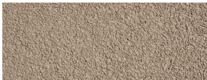
Exterior insulation and finishing system (EIFS)
