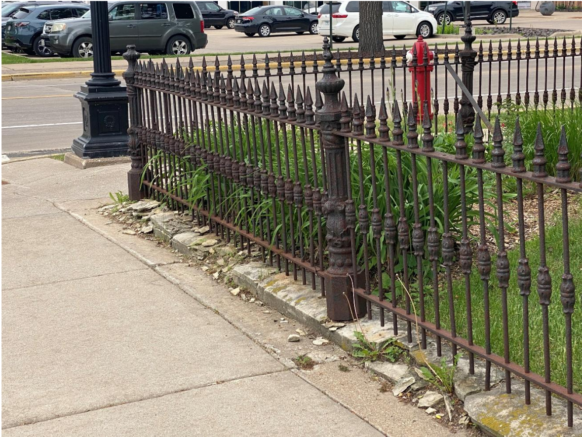
Existing Fence Condition:
