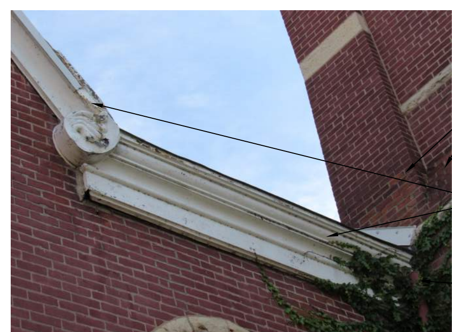
P3 METAL CORNICE NO SCALE
