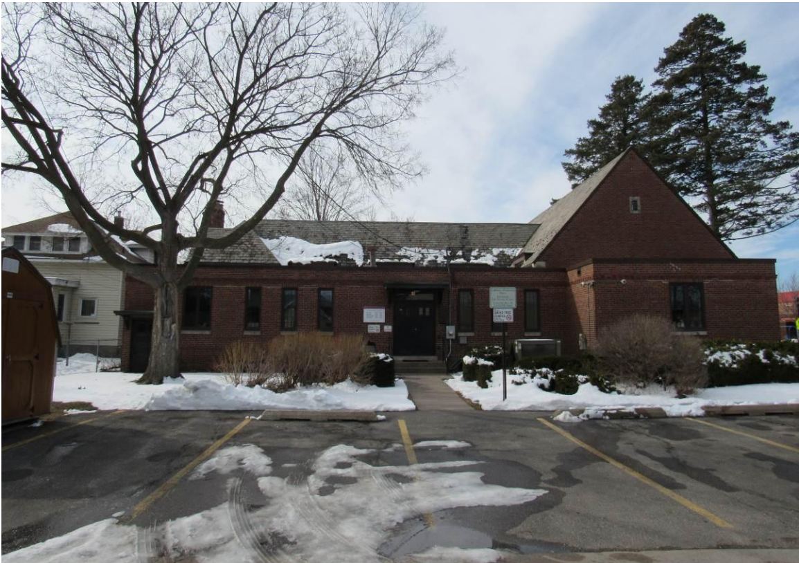
Figure 04 - East Elevation, North Community Library (2026).
