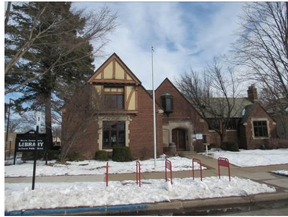
Figure 10 – Overall view of the west facade (2026).
