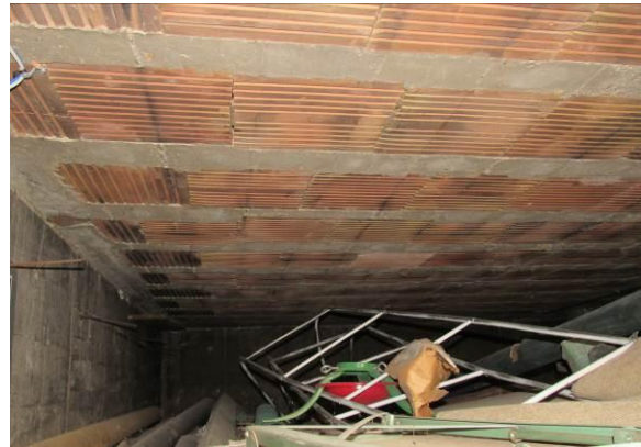
Figure 32 – Underside of concrete floor joist system (2026)
