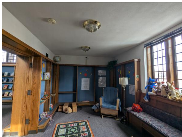
Figure 69 – Lighting in the north reading room of the Library (2026).
