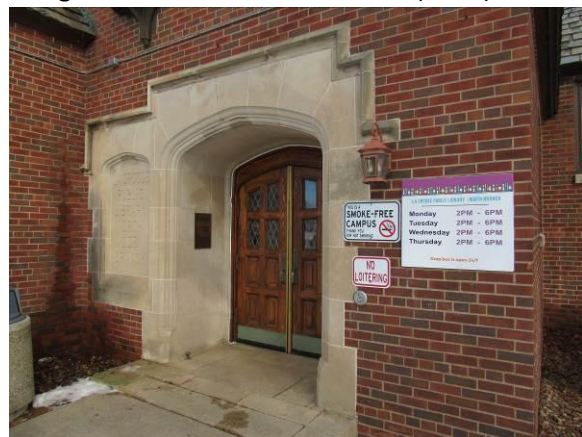
Figure 12 – Original front doors deeply recessed in the wall (2026).
