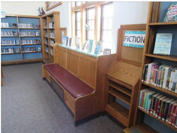
Figure 40 – Window benches double as duct chases (2026).
