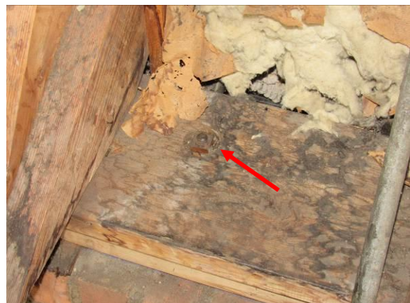
Figure 60 – Sill plates have anchor bolts embedded in the masonry below (2026).
