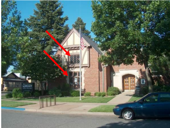
Figure 115 – The original windows were still extant until the 2007 window replacement project (2006).
