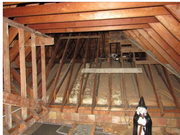
Figure 45 – Most of the attic has exposed roof structure with insulation below (2026).
