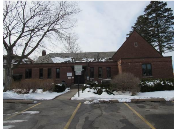
Figure 19 – Overall view of the east facade (2026).
