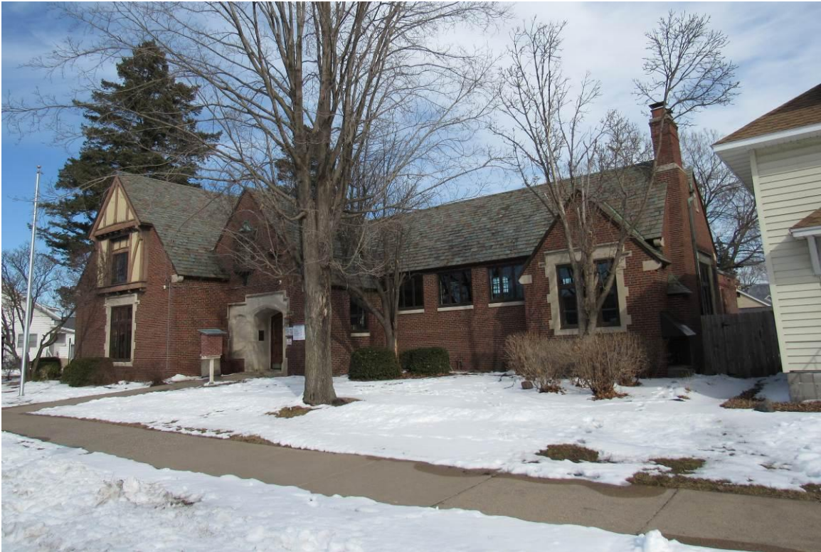
Figure 05 - South and West Elevations, North Community Library (2026).
