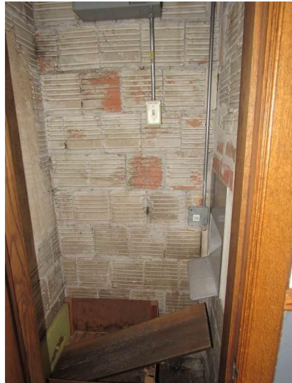
Figure 56 – The exterior masonry walls have an outside layer (wythe) of face brick and an inner layer(s) of hollow clay tile (2026).
