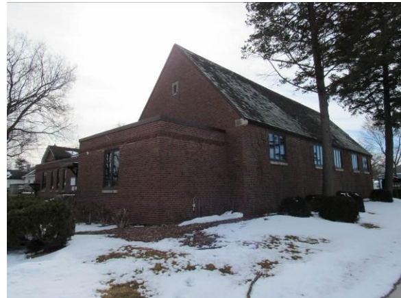
Figure 16 – Overall view of the north façade looking southwest (2026).
