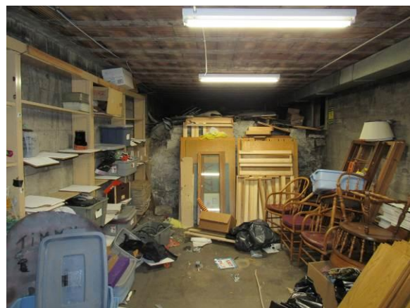
Figure 30 – North section of basement, notice old foundation wall & exposed concrete floor structure at ceiling (2026).
