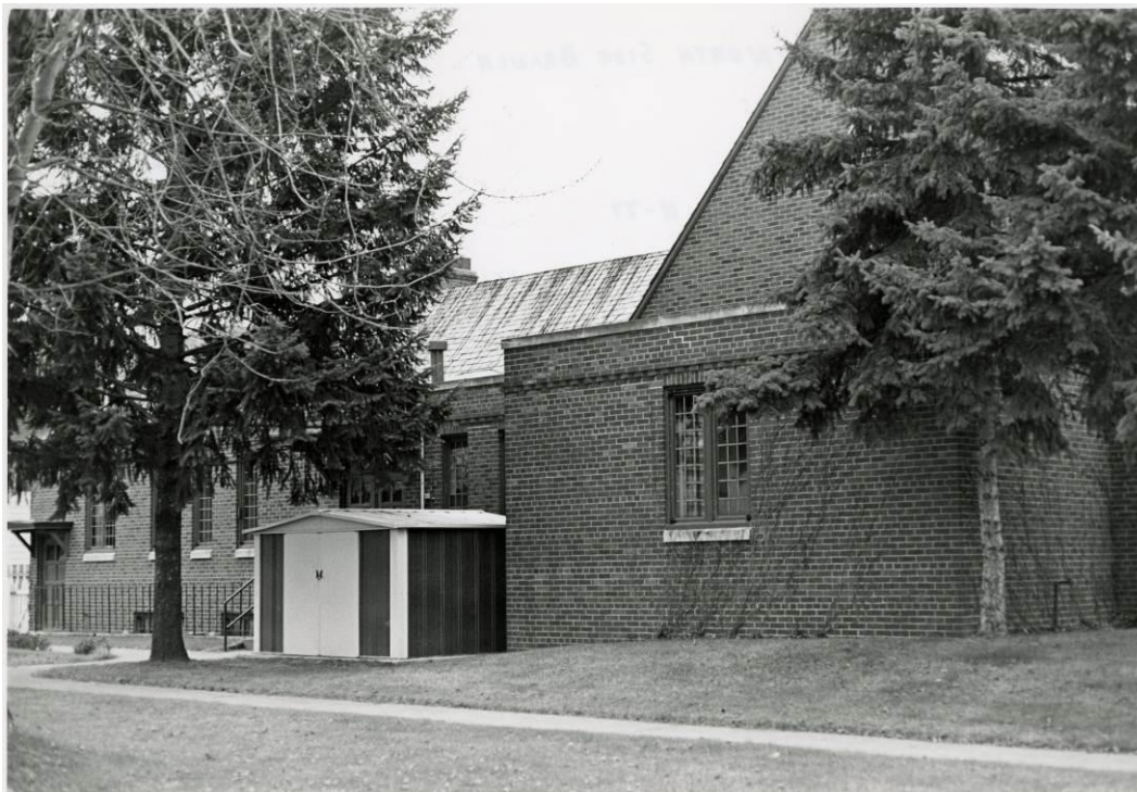
Figure 89 –View looking southwest at the back of the library. Circa 1977. Courtesy of the UW – La Crosse Murphy Library Special Collections.
