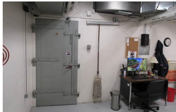
Figure 33 – Iron-clad door opening into mechanical room (2026).
