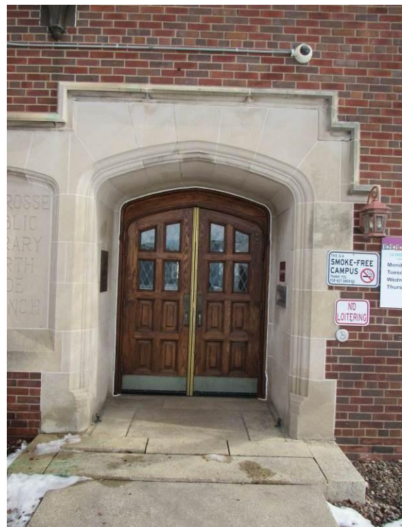
Figure 110 – The building has numerous security cameras, but they could have been installed to be more sympathetic to the architecture (2026).
