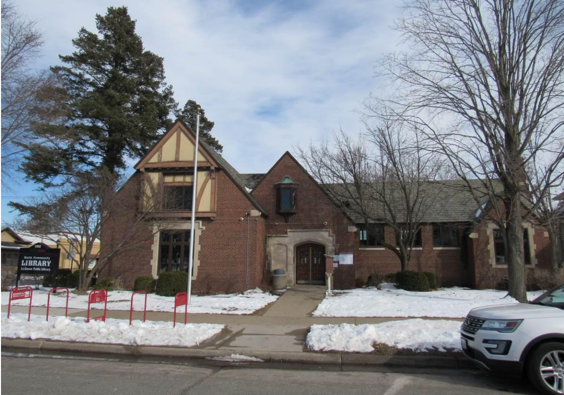
Figure 02 - West Elevation, North Community Library (2026).
