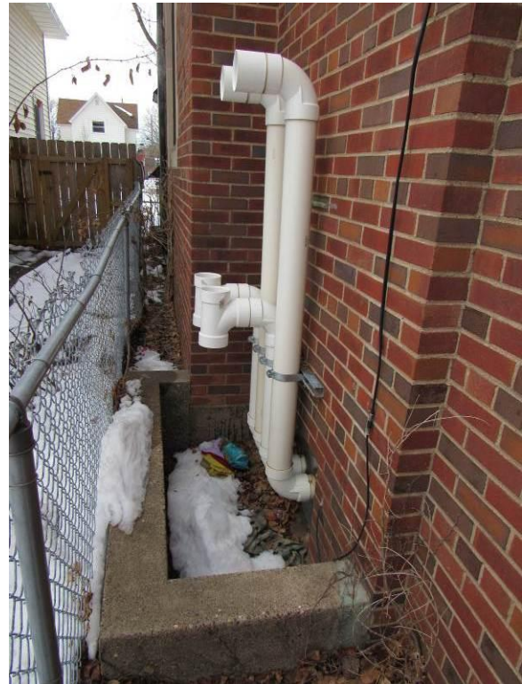
Figure 23 – Intake and exhaust for the HVAC are in a window well (2026).
