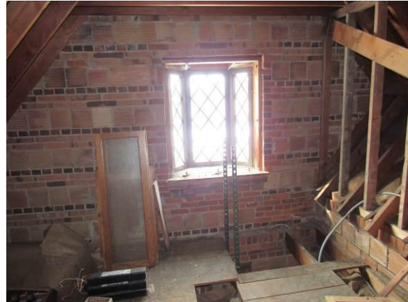
Figure 44 – The access scuttle is next to the oriel window (2026).
