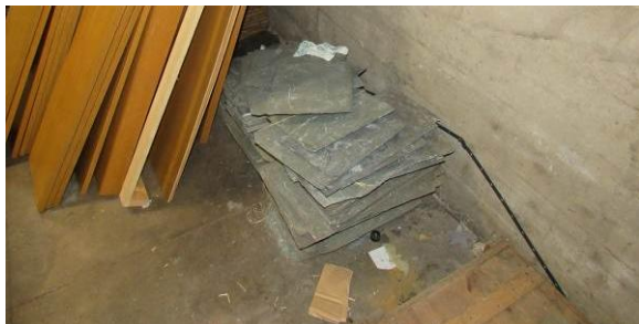
Figure 31 – Attic stock of slate roof shingles (2026).
