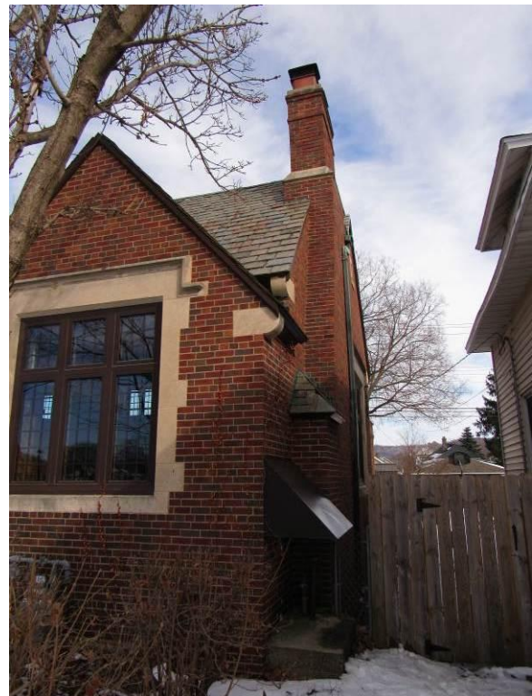
Figure 24 – The fence restricts access to the south facade (2026).
