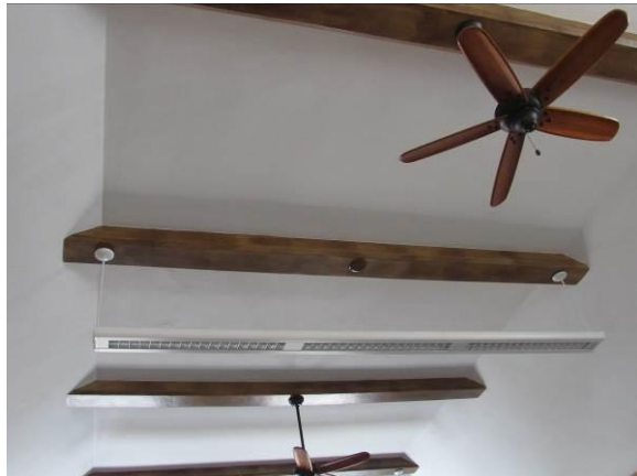
Figure 108 – Modern LED light fixtures and newer ceiling fans are in the main library space (2026).
