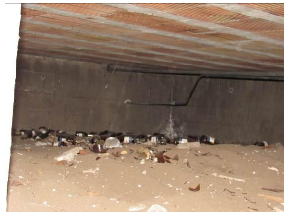
Figure 49 – Crawl space at the northwest corner of the basement (2026).
