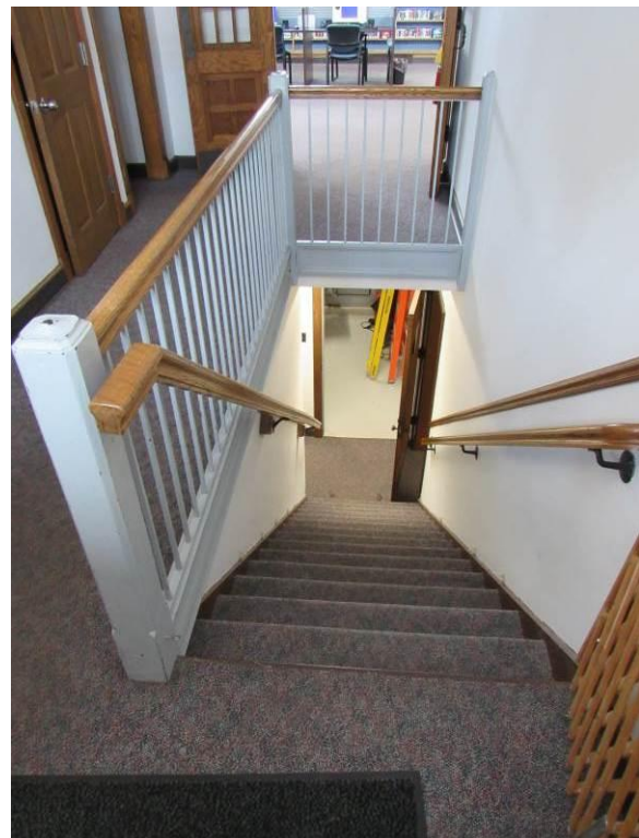
Figure 39 – Steel stairs to the basement meeting rooms and mechanical (2026).
