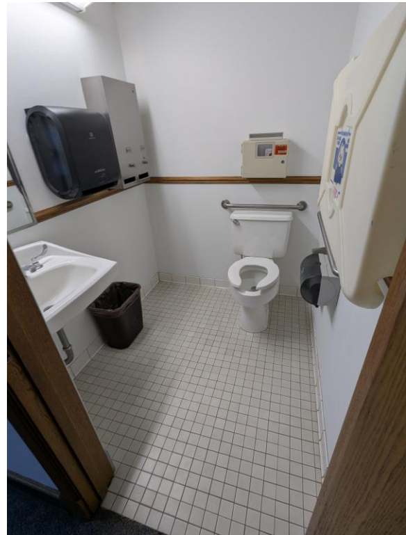
Figure 76 – Main Level Public Toilet Room (2026).
