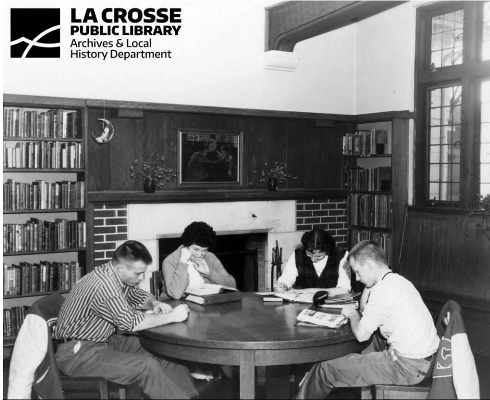
Figure 84 – View looking at fireplace in main library. Date Unknown. Courtesy of La Crosse Public Library Archives.
