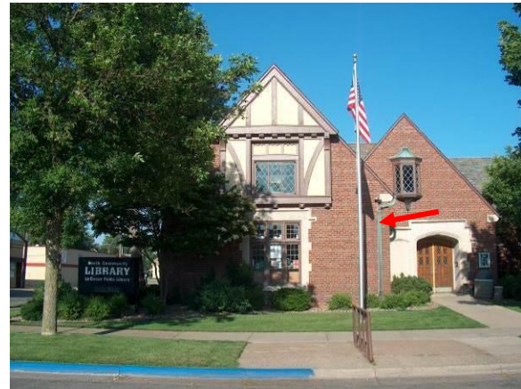
Figure 103 – The building originally had copper gutters and downspouts (2006).
