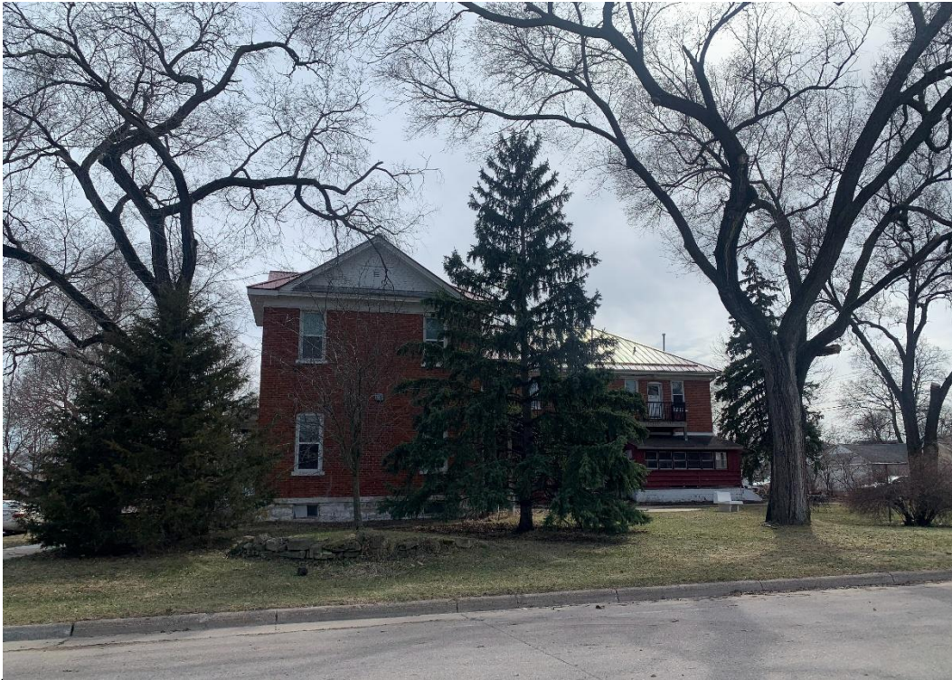
Figure 22 – View of the north façade of the Goddard Hotel. March 2026.
