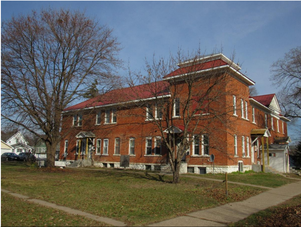
Figure 16 – View of the south façade of the Goddard Hotel. March 2026.
