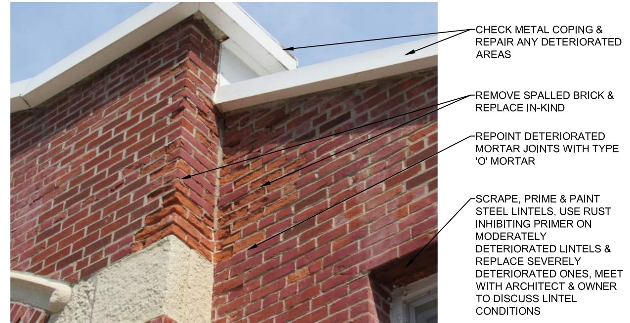
P3 SPALLED BRICK NO SCALE
