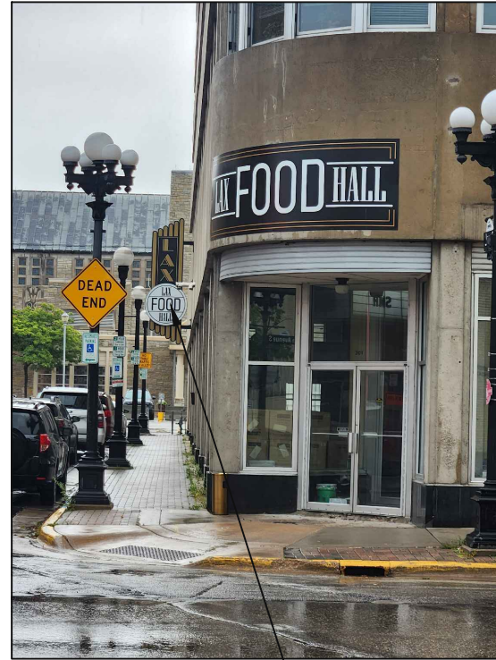
PROPOSED HOOD DUCT EXHAUST FANS WILL BE HIDDEN BY EXISTING SIGN FROM VIEW FROM 5TH AVE
