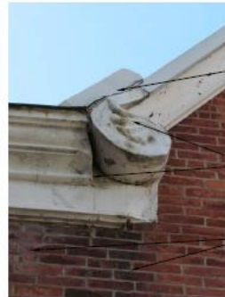
P6 CORNICE DETERIORATION NO SCALE
