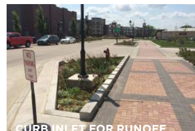
CURB INLET FOR RUNOFF
