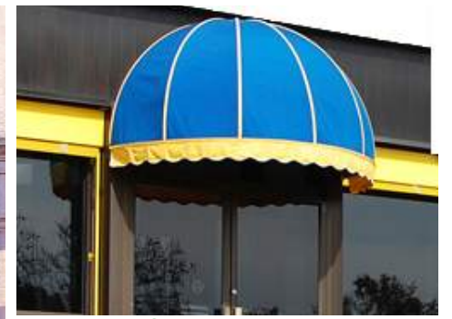
Example of Unacceptable Awning
