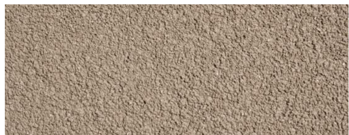
66 Exterior insulation and finishing system (EIFS)
