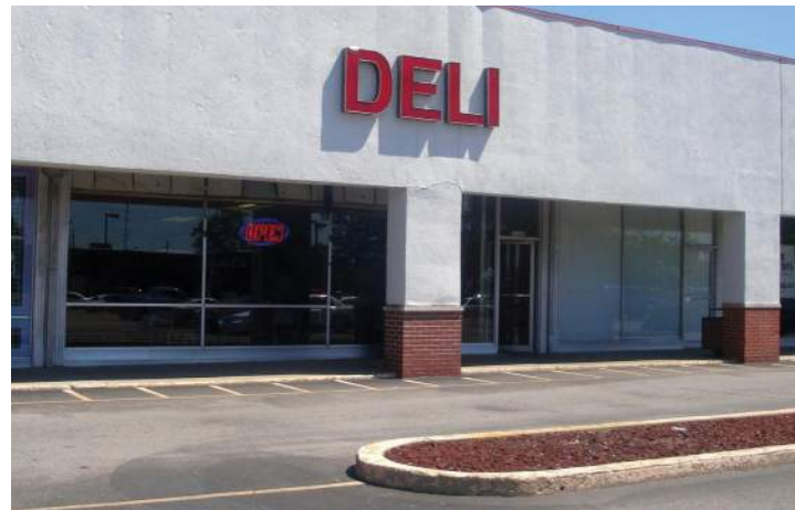
Unacceptable Signage Placement
